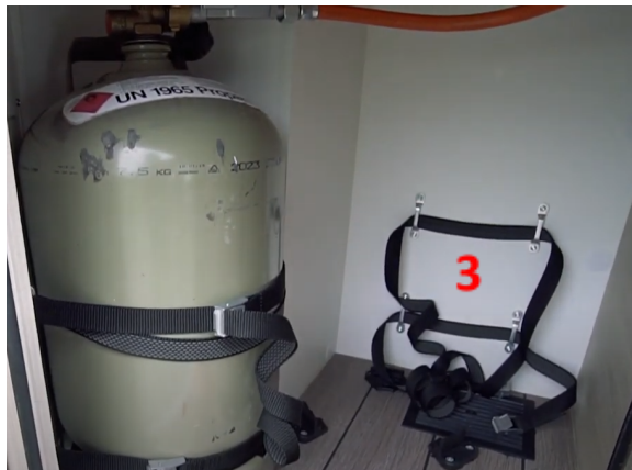
Fig. 4.1 - Gas cylinder installation
